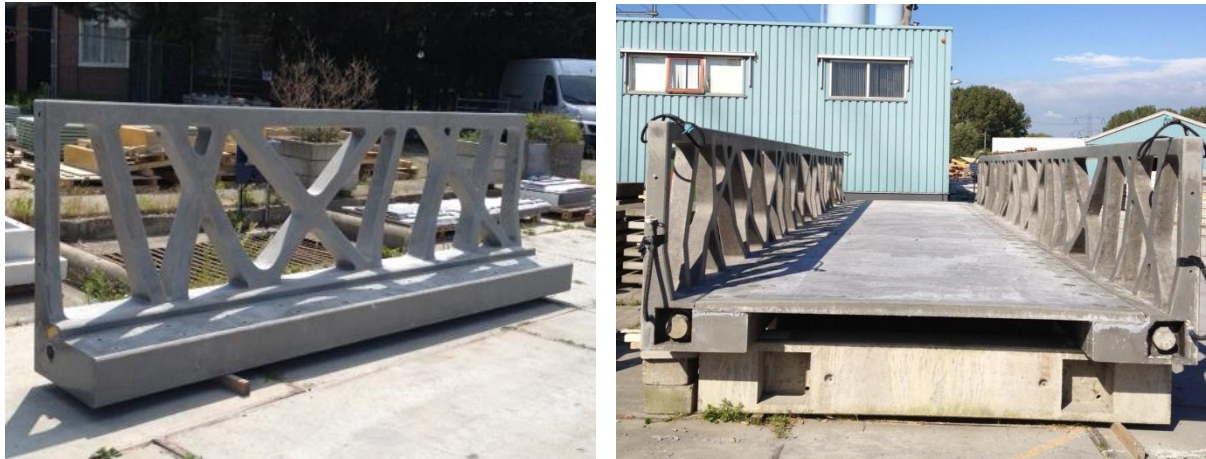
Figure 4: The 4.3m long handrail element (left), connected and pre-stressed elements (right)
