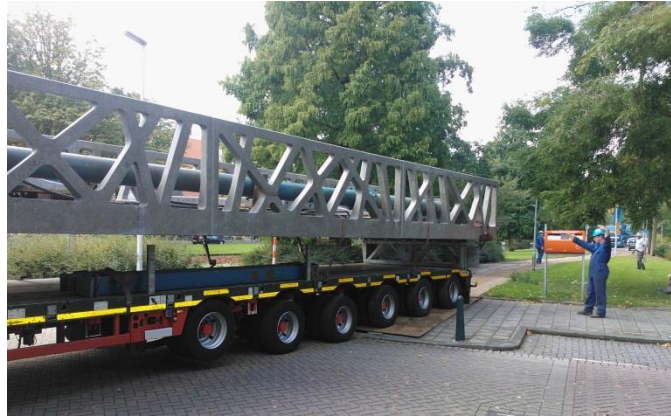
Figure 6: Transport of the bridge to the definite location
