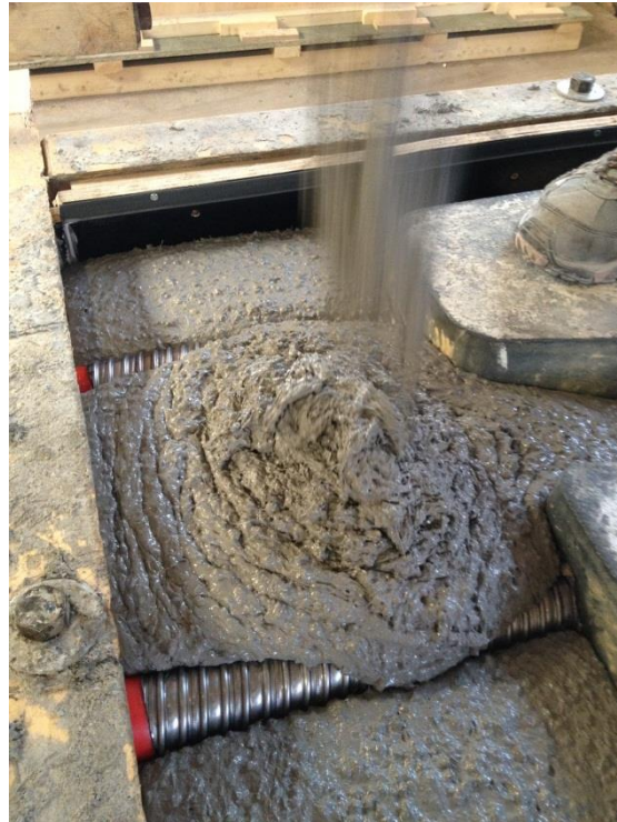
Figure 5: Low w/c ratio makes the concrete thixotropic
